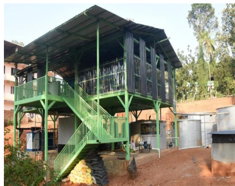
1 MLD STP at Kozhikode medical College
